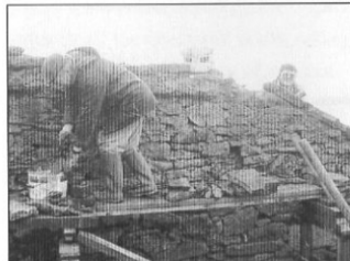
Ian Girvan supervising Bill Carty hard at work pointing the wall.
