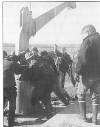
Installing new crane on site.
